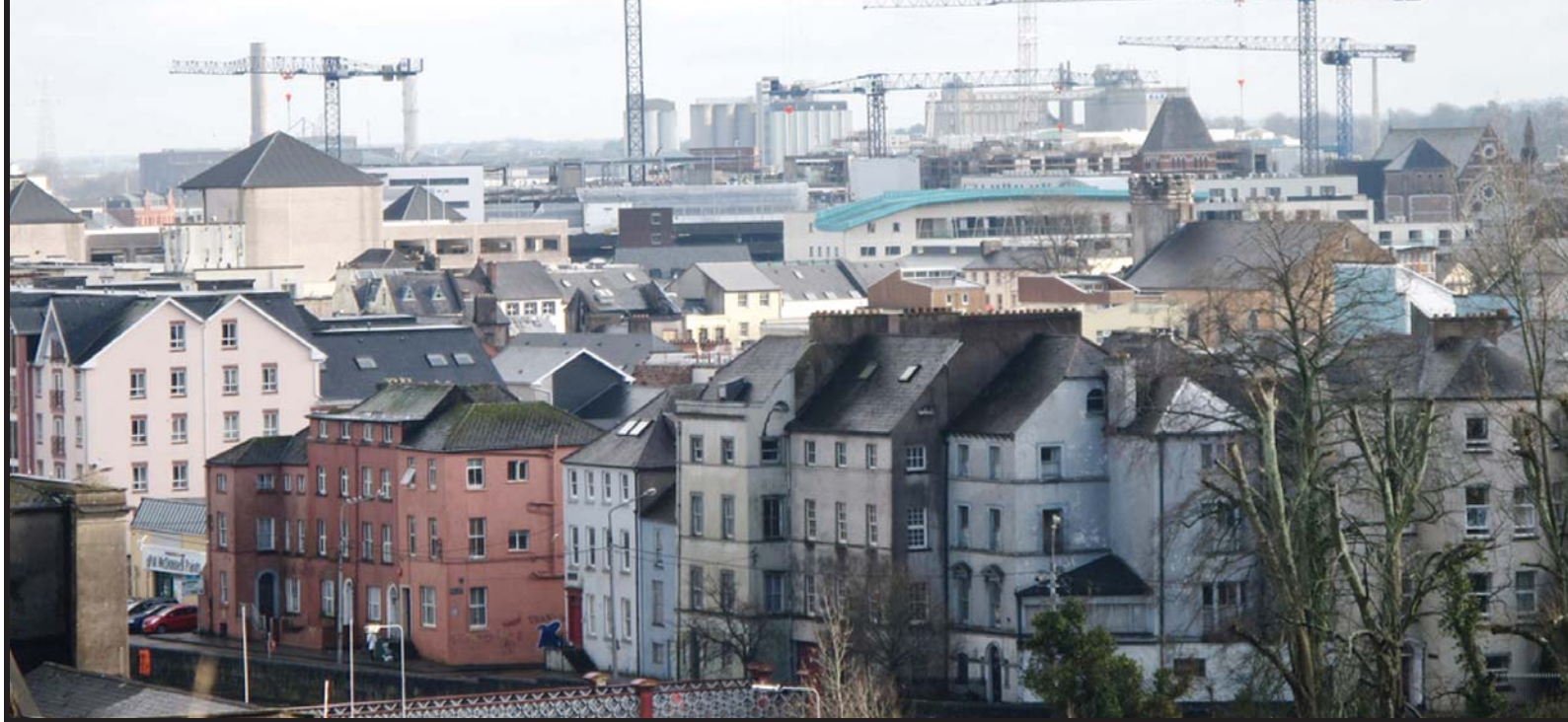
Construction work in Cork city during the boom years
